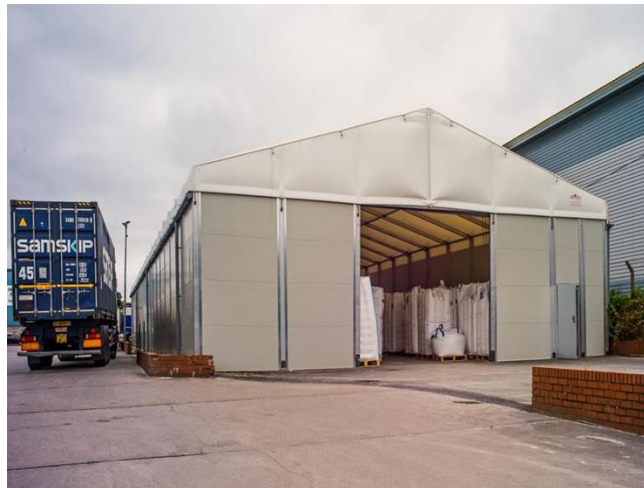
Example-Fabric Covered Structure
