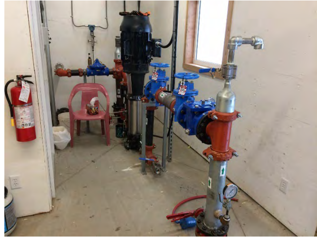
Figure 5: Example of a 50hp multi-stage vertically stacked pump
