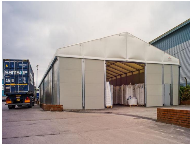
Example-Fabric Covered Structure
