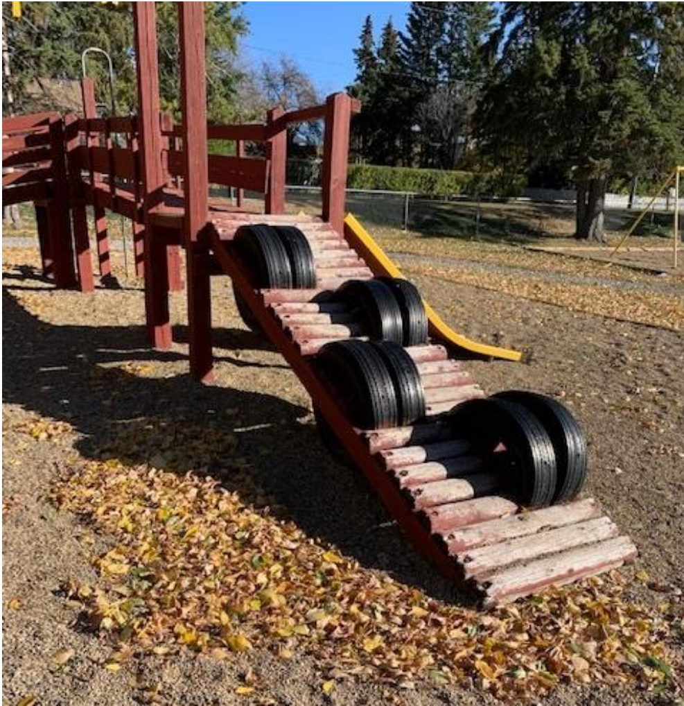
This ramp requires handrails along each side
