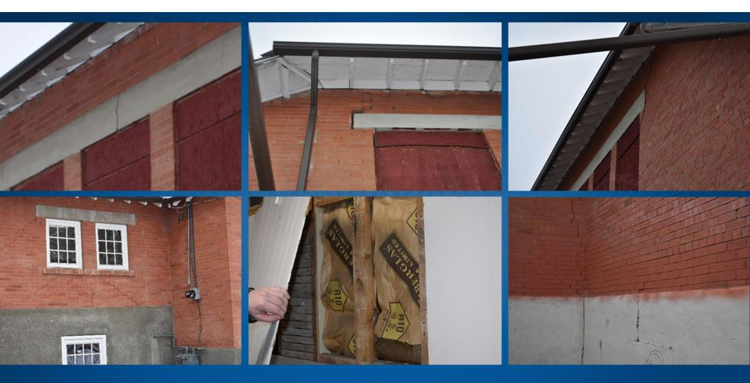
Roof Framing and Load Bearing Brick Walls
